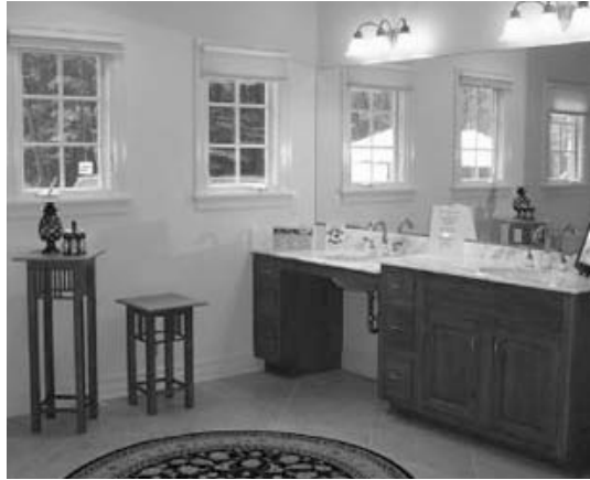
Example of ample maneuvering clearance, lowered sink with knee clearance and proper lighting.
