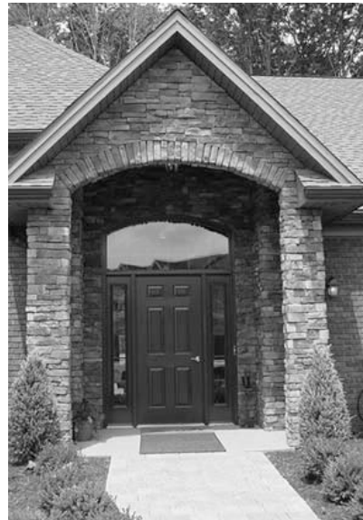
Example of a no-step, or barrier-free, entryway
